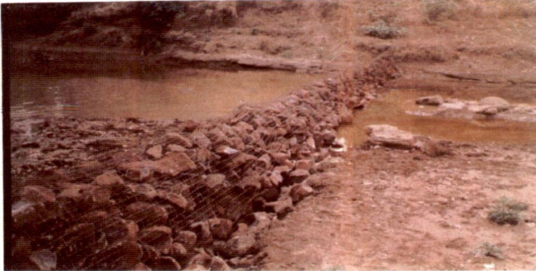
Fig.4.2 Schematics of a Gabion Structure
