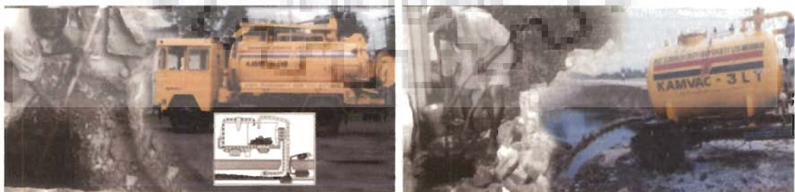
Fig. 7.11: The traditional way vs the recommended way of cleaning drain silt
