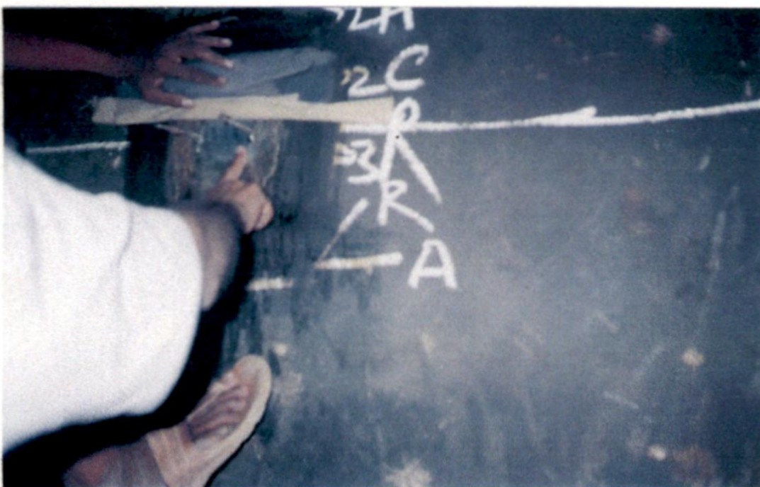
Application of araldite for proper bonding
