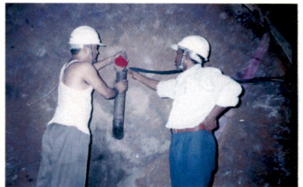
Pipe bend was filled with epoxy
