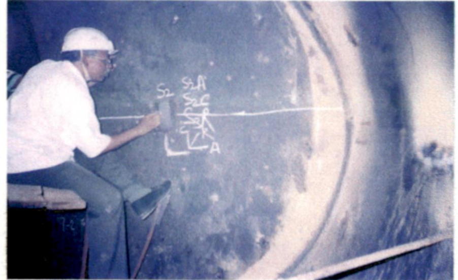
Cleaning of surface area of size 100mm x 100mm
