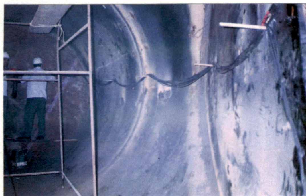
Cable routing through pipe bend for internal gauges
