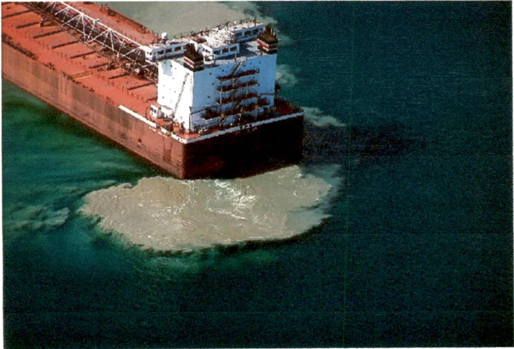
FIG.2 PICTURE SHOWING OPEN WATER DISPOSAL OF DREDGED MATERIAL
