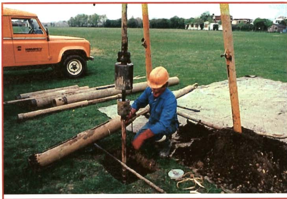
Plate 4.2 Standard Penetration Test (SPT) in Progress
