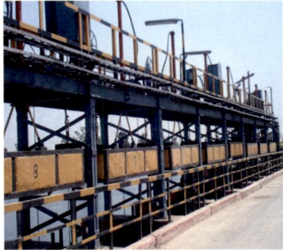
Intake gates at Salar SHP
