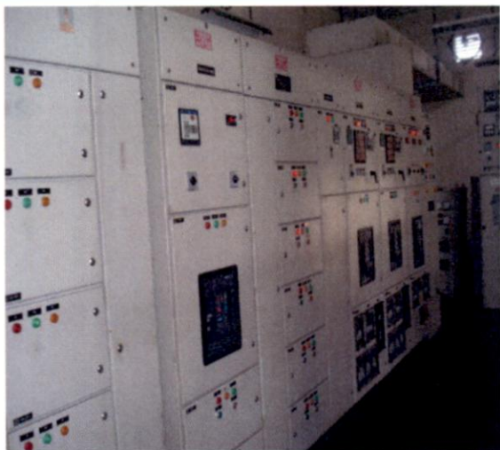
Protection panels at Babbanpur SHP
