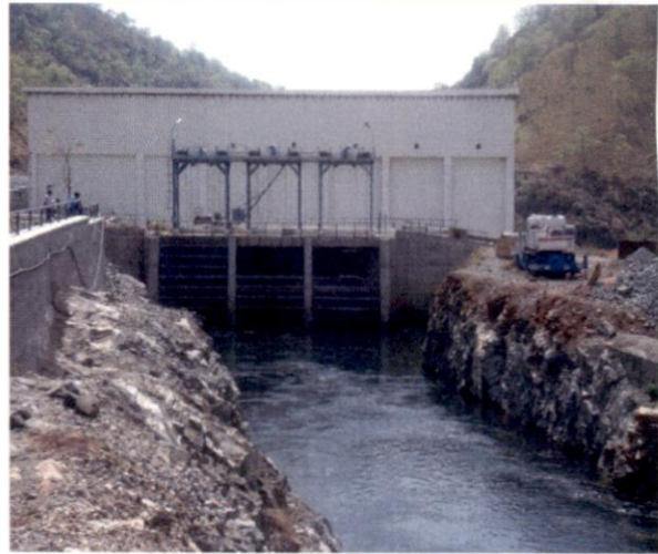
Intake gates at Someshwara SHP
