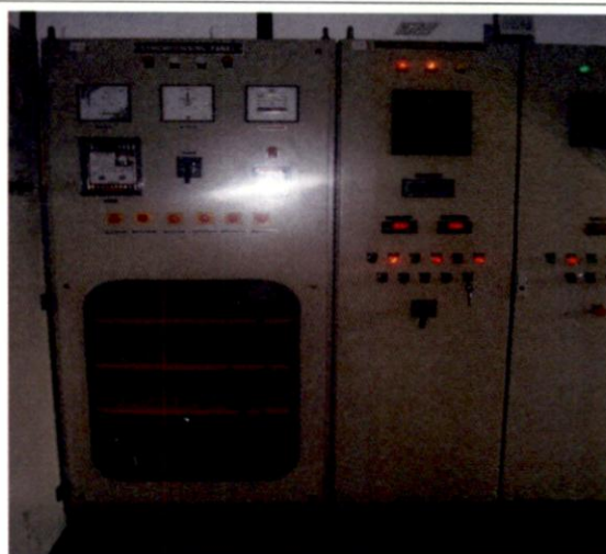
Synchronization and line panel at Ranganathaswamy SHP
