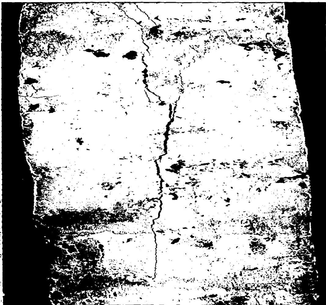
Plate 4 Crack pattern in plain column
