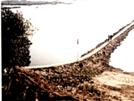
Construction of river training structures to achieve adequate water depth
