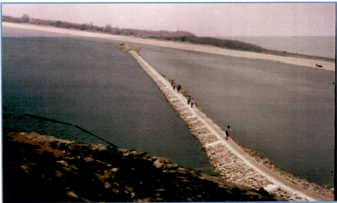
Fig 6.5 Impermeable Groyne
