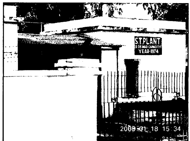
STP at Durgapur industrial colony
