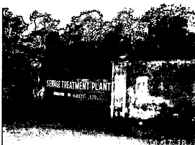
STP of Durgapur Project Ltd.
